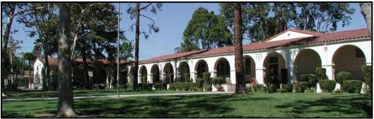
Figure 12. Reseda Elementary School, 1936. The spare Mission Revival style was in keeping with the post-Field Act requirement for one-story massing and the post–Long Beach Earthquake trend to design in the "traditional Southern Californian" mode. Source: LAUSD.
